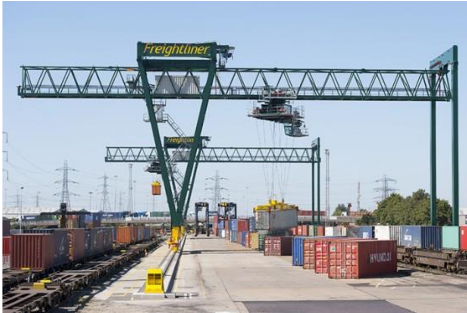
Figure 4.2 - Gantry Cranes Operating in a UK Railport
